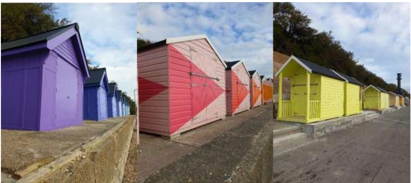
New and renovated beach chalets painted with Rana Begum's colourful design.
