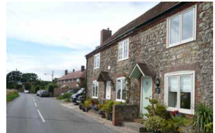
Local Greensand and Kentish Ragstone in the older buildings of Lympne, Aldington and Westenhangar
