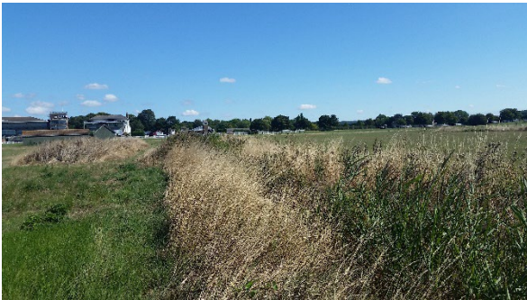
TN20 – 600m of ditches
