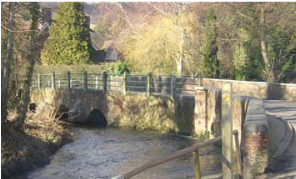
The route into Shoreham
