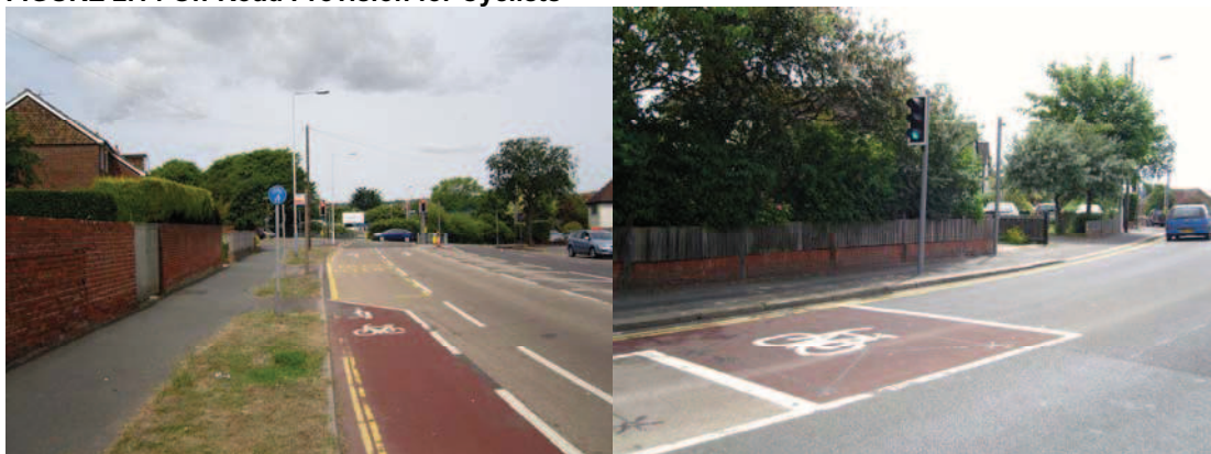
FIGURE 2.14 On-Road Provision for Cyclists
