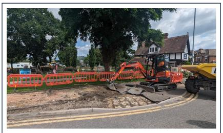
Here we are breaking out redundant footways by Radnor Park roundabout, these will be replaced with new materials.
