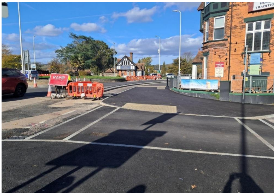
Improved junction works at Radnor Park roundabout.
