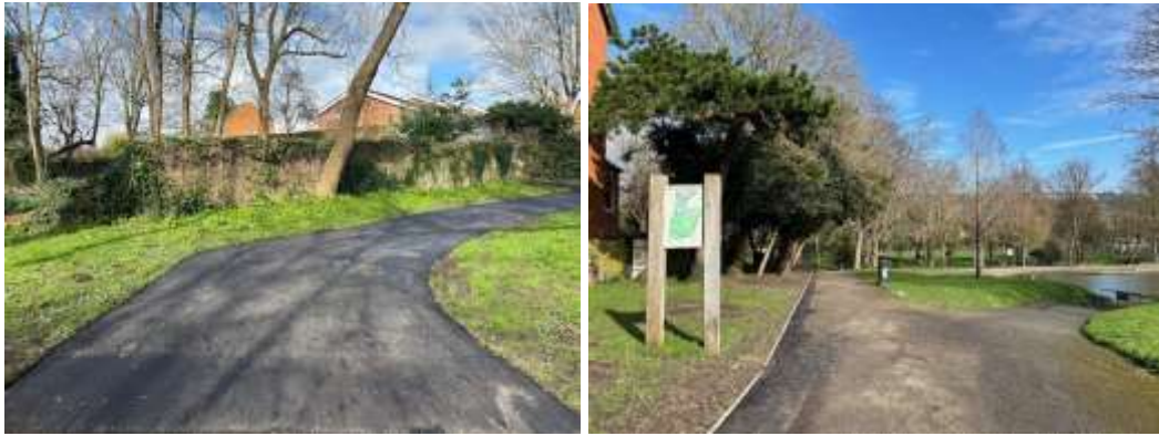
Infrastructure improvements April 2024
