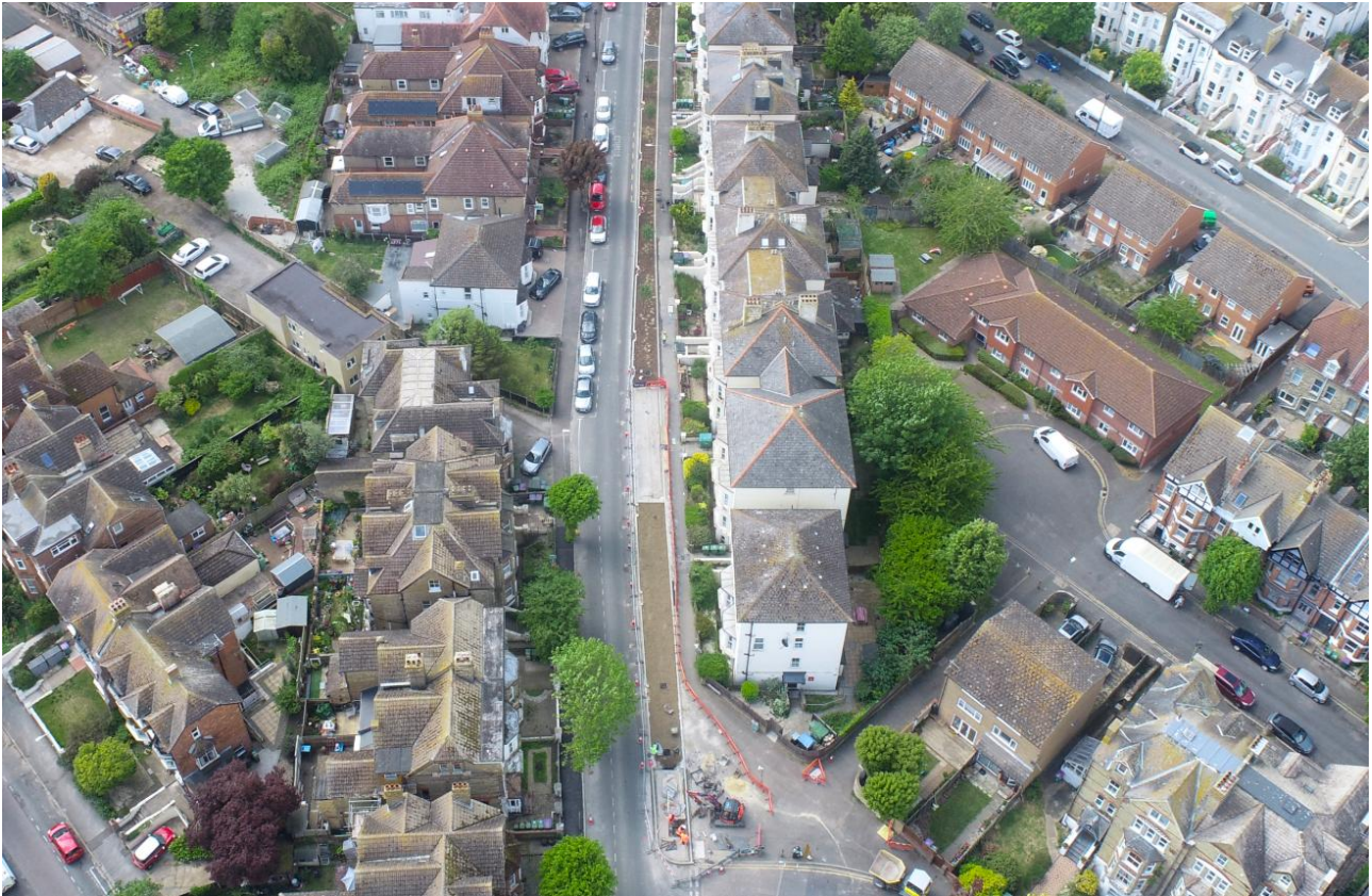
Cheriton Road / Connaught Road works
