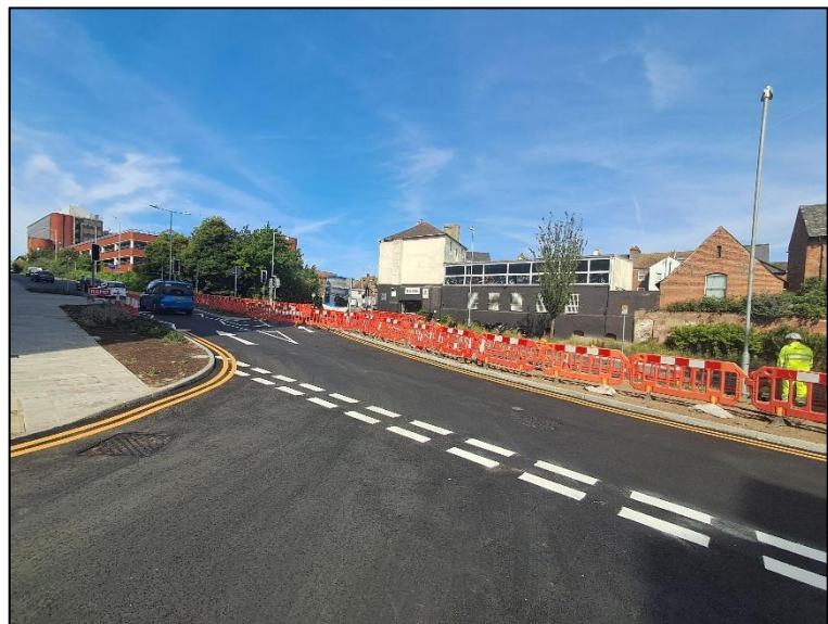
Resurfaced Road and New Road Markings; Shellons Street / Entrance of Gloucester Place
