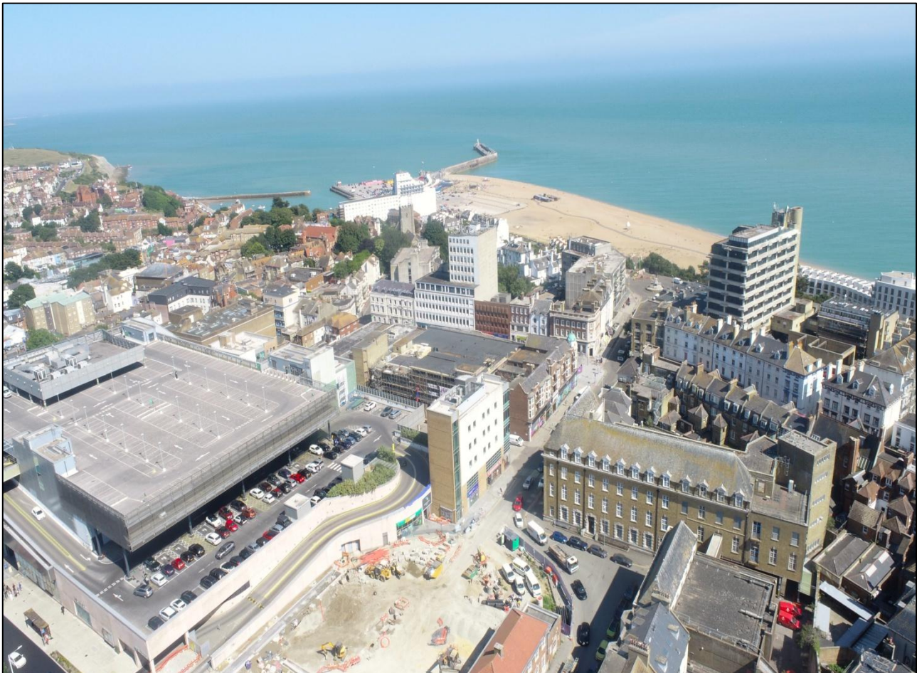
Aerial view of Folkestone Town Centre.
