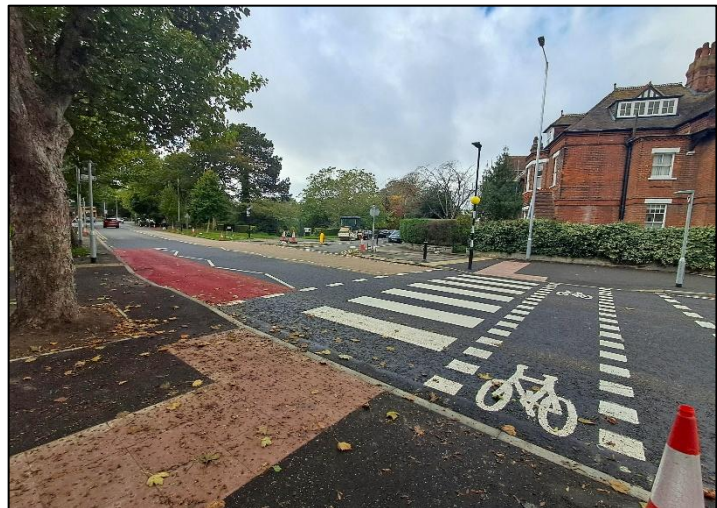
Newly constructed crossing – Station Approach
